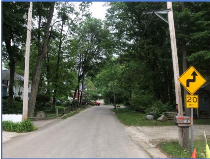
Photo 69: Very tight limits with low sight distance. OHE poles on north side and OHT on south, both 2' from EOP.
