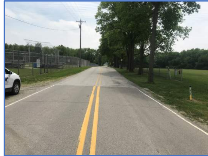
Photo 6: East fence 12' from EOP. West fence 15' from EOP. 3Ph OHE on east side, 10' from EOP. Gas, fiber, and water on west side. Gas at EOP, other west utilities behind fence.
