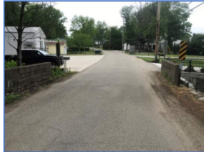
Photo 62: Existing Small Structure Reinforced Concrete Slab (Asset No.: 43-0014-00000-25) Max Span Length (ft): 9.0; Length Along Skew (ft): 26.0; Height of Opening (ft): 4.4
