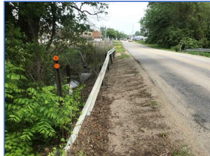
Photo 20: Guardrail offset 6' from EOP with unstable gravel shoulder 2:1 slope. CMP may need extended for trail.
