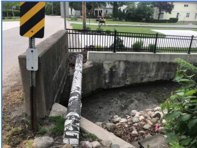
Photo 63: Existing small structure with gas main exposed.
