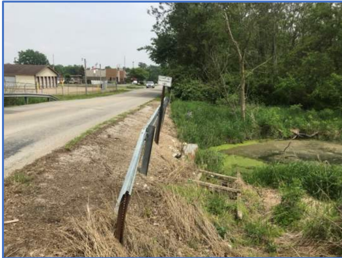
Photo 21: Guardrail with unstable gravel shoulder.
