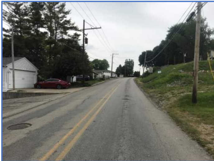
Photo 75: Steep embankment on south and OHE pole set 5' from EOP on north. Limited sight distances throughout.
