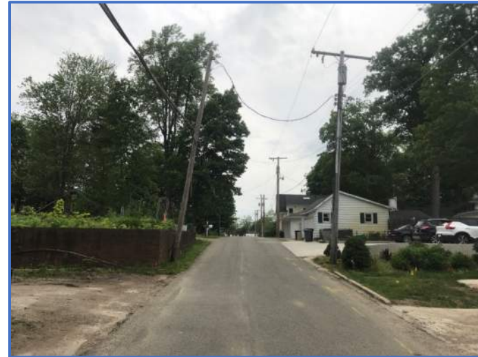
Photo 70: Very tight limits with low sight distance. OHE poles on north side and OHT on south, both 2' from EOP.
