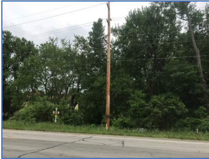
Photo 53: NIPSCO 69kv transmission with apparent UG comm on south side of SR 13.
