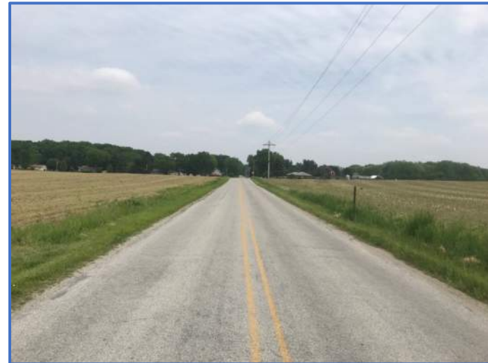
Photo 12: OHE and fiber on south side of E 1200 N. Poles offset 5' from EOP from Kern Rd. to Syracuse Webster Rd.
