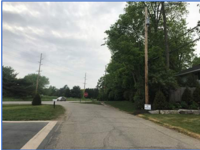
Photo 61: At intersection of Southshore Dr. and SR 13. NIPSCO OHE with comm under build on north side (waterfront side).
