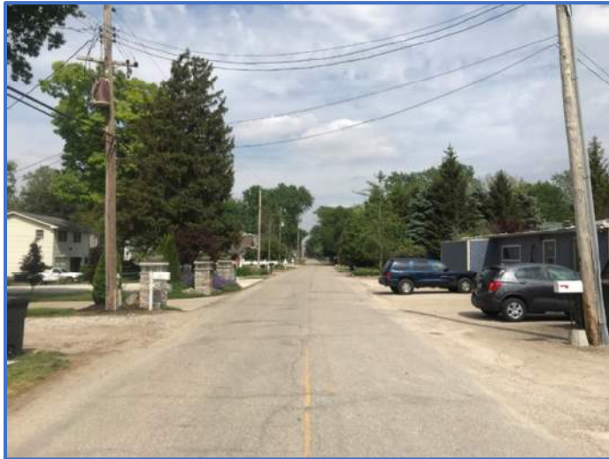
Photo 45: OHE with comm under build along north side of Waco Dr.
