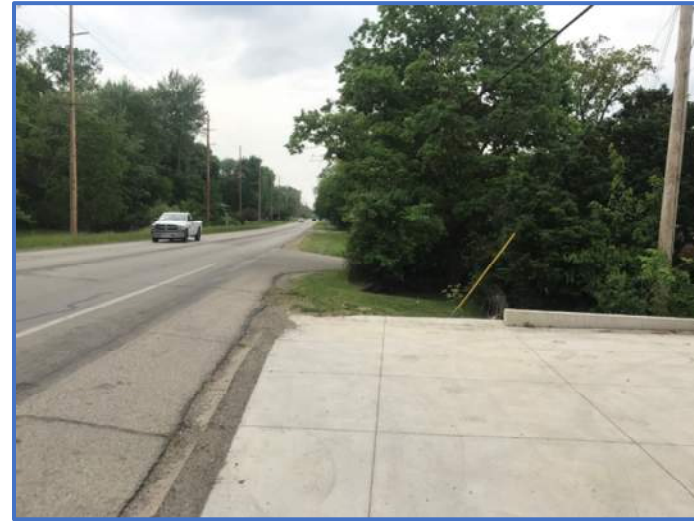
Photo 54: North side of SR 13, 10' wide paved shoulder. Drive pipes and mailboxes throughout. Gas pipeline markers near mailboxes.
