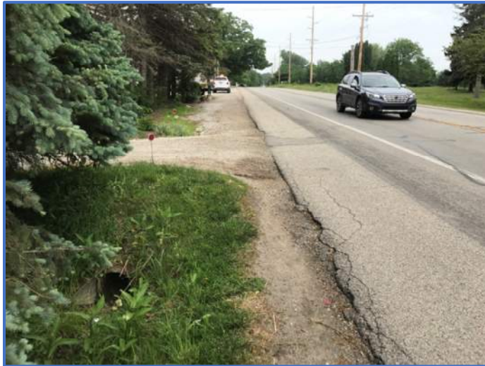
Photo 57: North side of SR 13, 10' wide paved shoulder.
