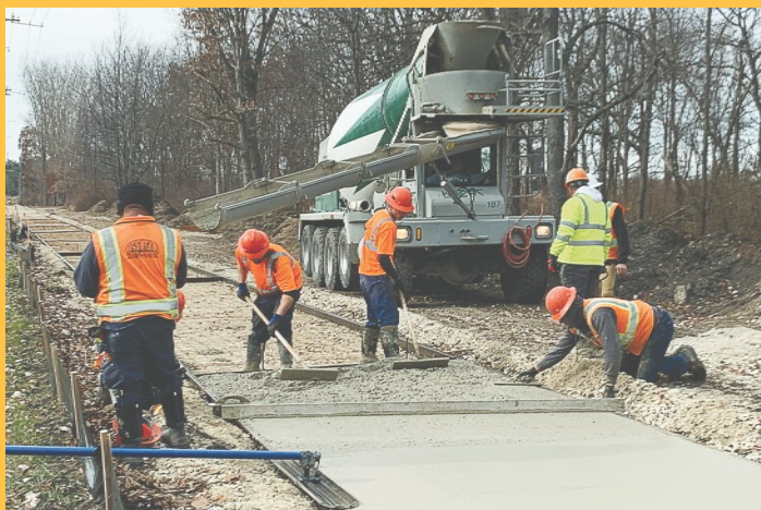
Starting concrete work.
