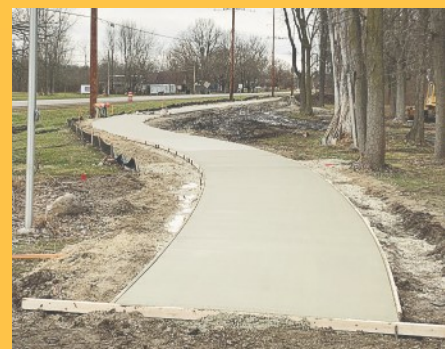
Conklin 1st cement segment completed on Dec. 2, 2019.
