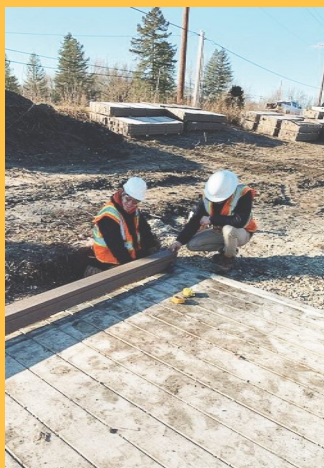
Boardwalk in progress.
